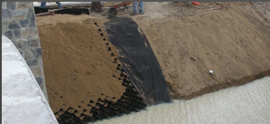
EnviroGrid® Geocell Infilled with Native Sandy Soil
