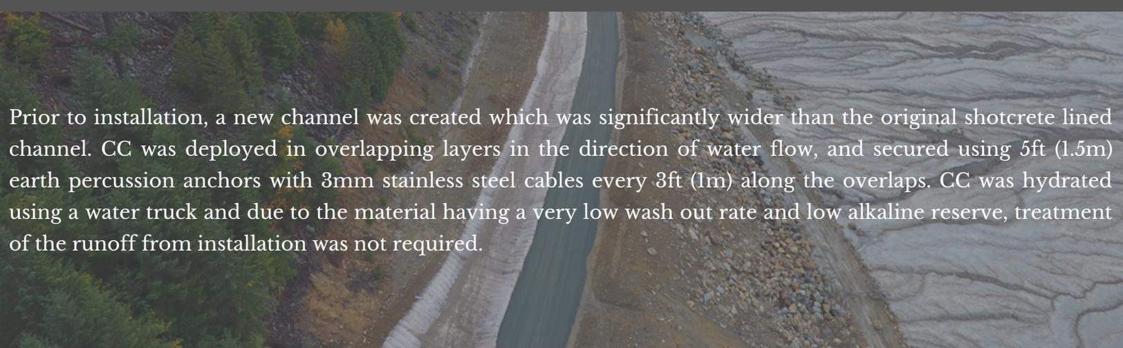
Prior to installation, a new channel was created which was significantly wider than the original shotcrete lined channel. CC was deployed in overlapping layers in the direction of water flow, and secured using 5ft (1.5m) earth percussion anchors with 3mm stainless steel cables every 3ft (1m) along the overlaps. CC was hydrated using a water truck and due to the material having a very low wash out rate and low alkaline reserve, treatment of the runoff from installation was not required.
