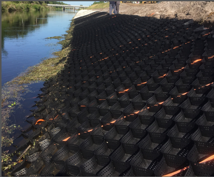
EnviroGrid® Geocell with 2,200LB Tendon
