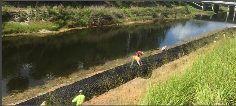
Installation of EnviroGrid® Geocell Layer
