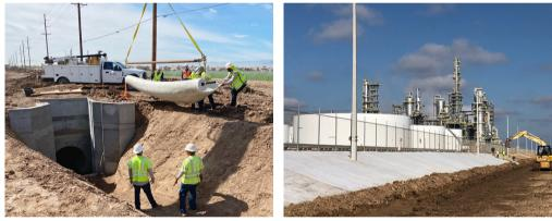
Reinforced Concrete Roll<sup>®</sup> is a dry powdered concrete that is needle-punched between two pieces of non-woven, polypropylene. When rolled out and hydrated, it takes shape into a durable structure suitable for reinforcement or protective lining.
