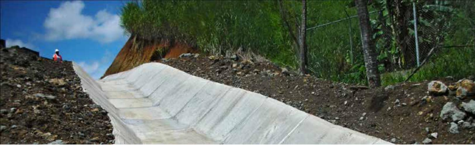
**Concrete Infilled Channel**
